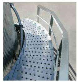
**Optional sidewall ladders** (right) and BROCK SHUR-STEP® Bin Stairs (above), as well as safety cages and rest platforms, conform to OSHA standards and are fabricated from galvanized steel for long-lasting service.
